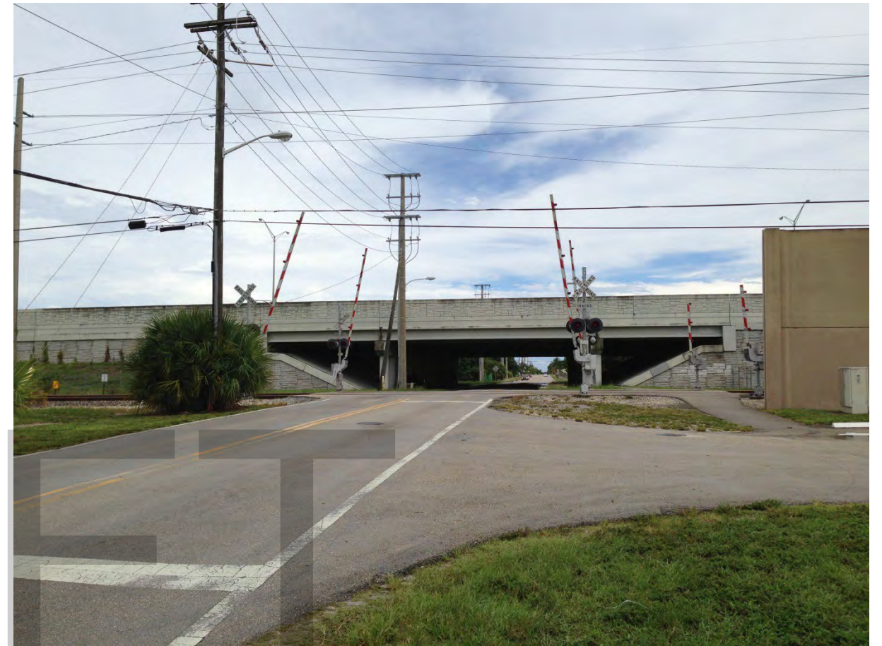
Example of 4 Quadrant Gate Installation:
