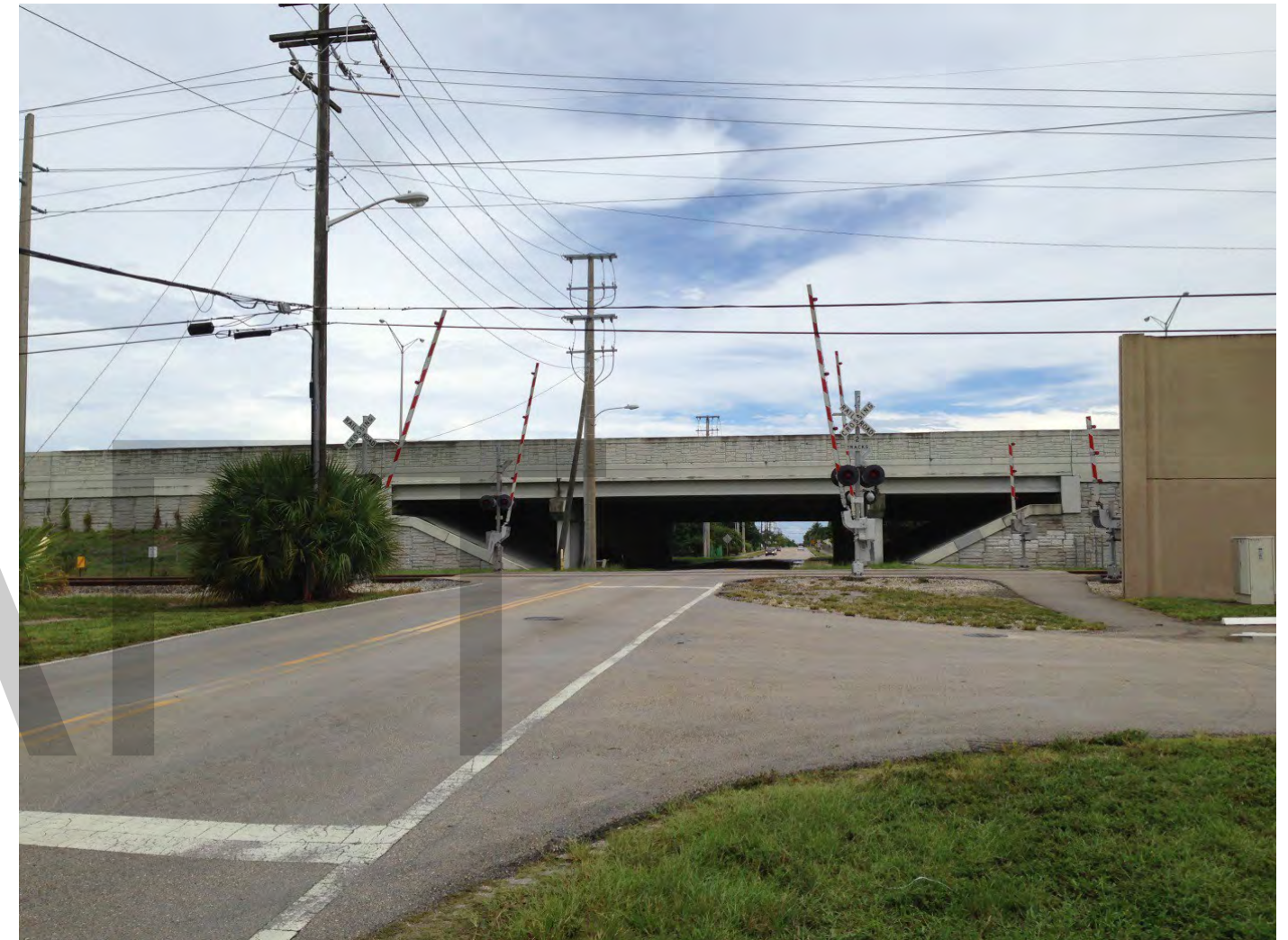
Example of 4 Quadrant Gate Installation:
