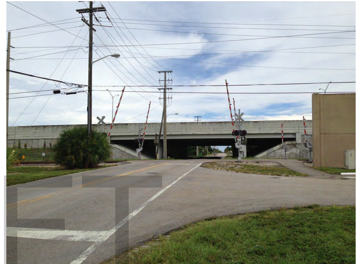
Example of 4 Quadrant Gate Installation:
