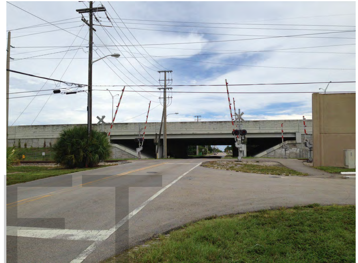
Example of 4 Quadrant Gate Installation:
