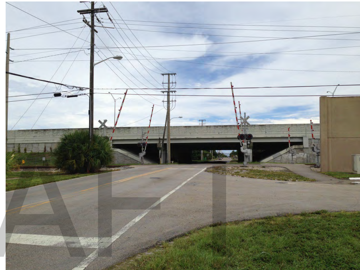
Example of 4 Quadrant Gate Installation:
