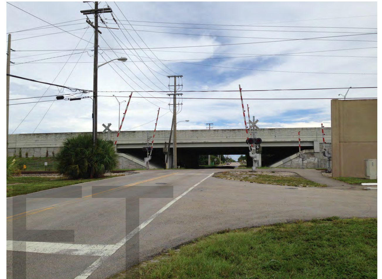
Example of 4 Quadrant Gate Installation:
